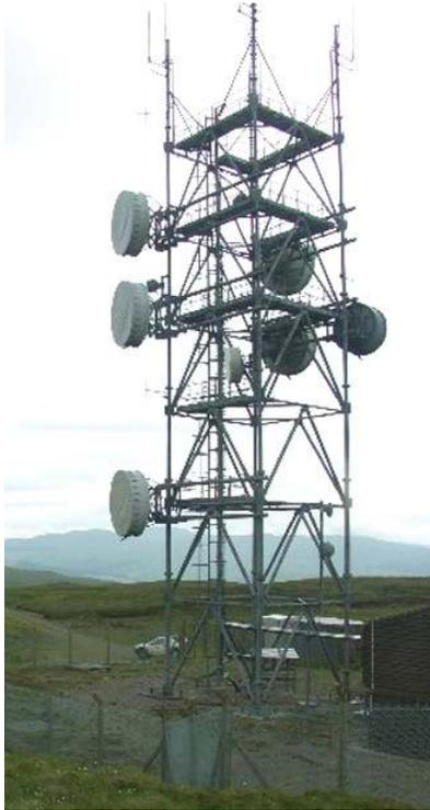
Figure 6a. Microwave repeater showing multiple co-located antennas.[3]
